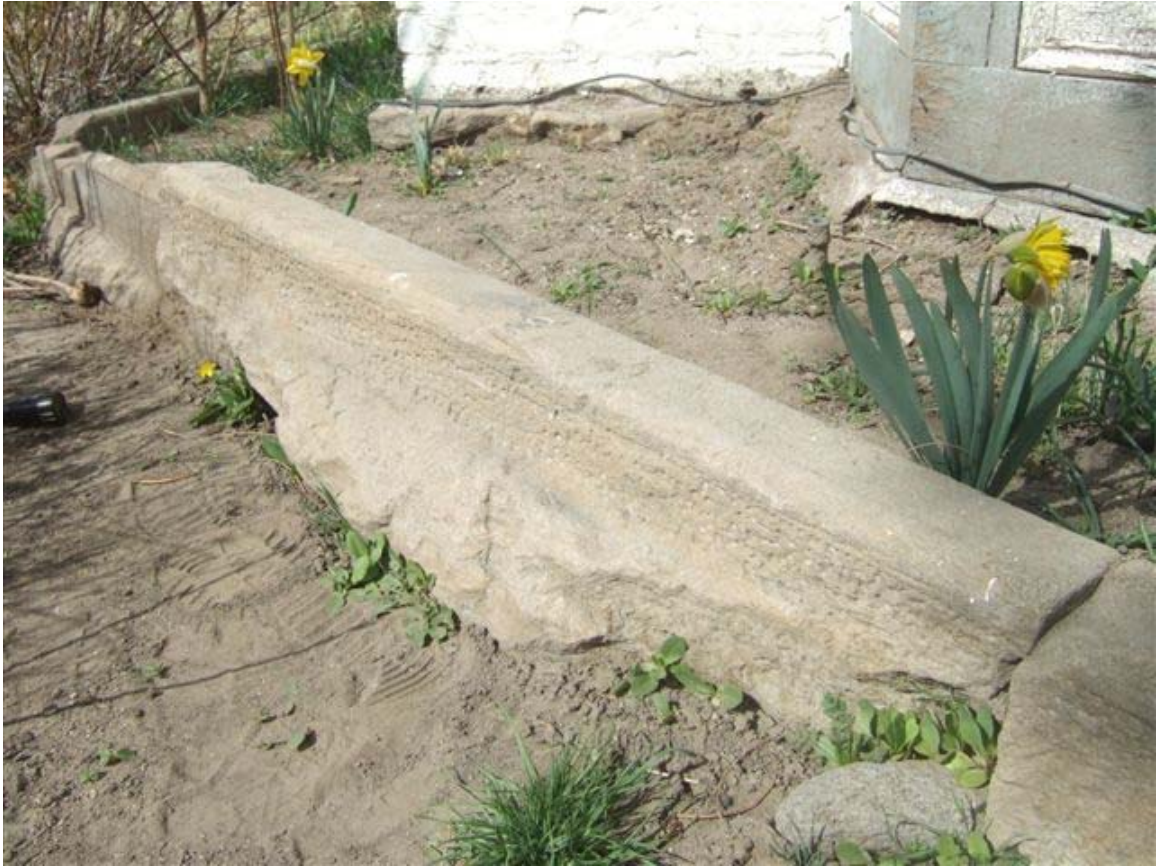
3. The Rectory's stone walkway and flower bed borders were probably added during the Hatch years.
