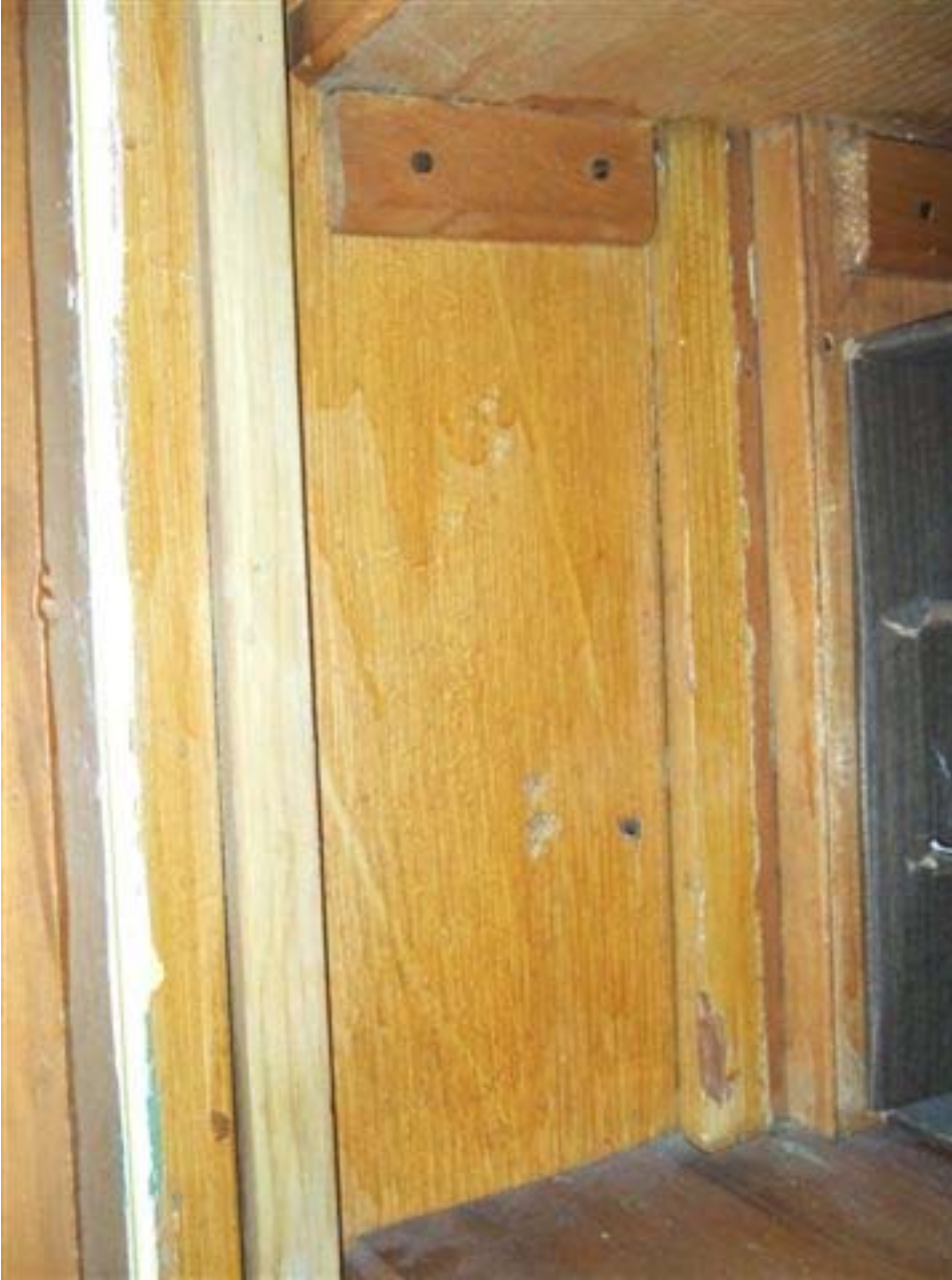
19. Graining in the built-in cabinet of the side wing.
