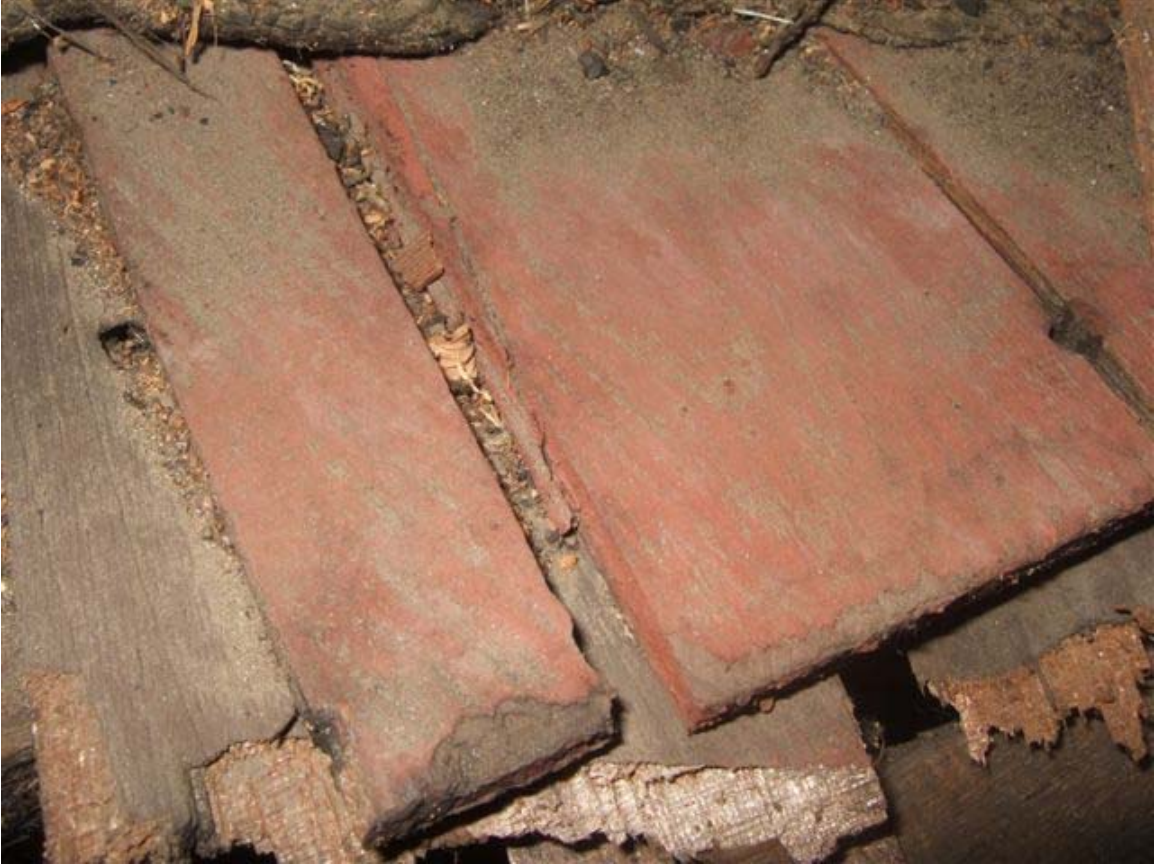
11. Red-painted wood roof shingles preserved in the attic.
