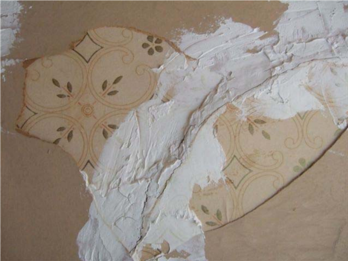
17. Wallpaper in the upstairs storeroom.
