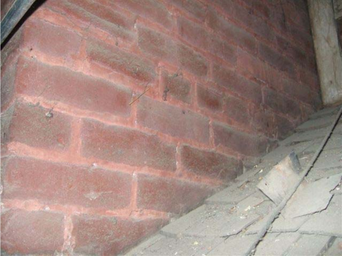
12. Red oxide wash visible in the attic.
