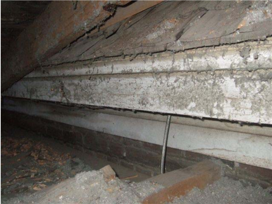
13. Formerly exterior west (rear) elevation cornice of the side wing.
