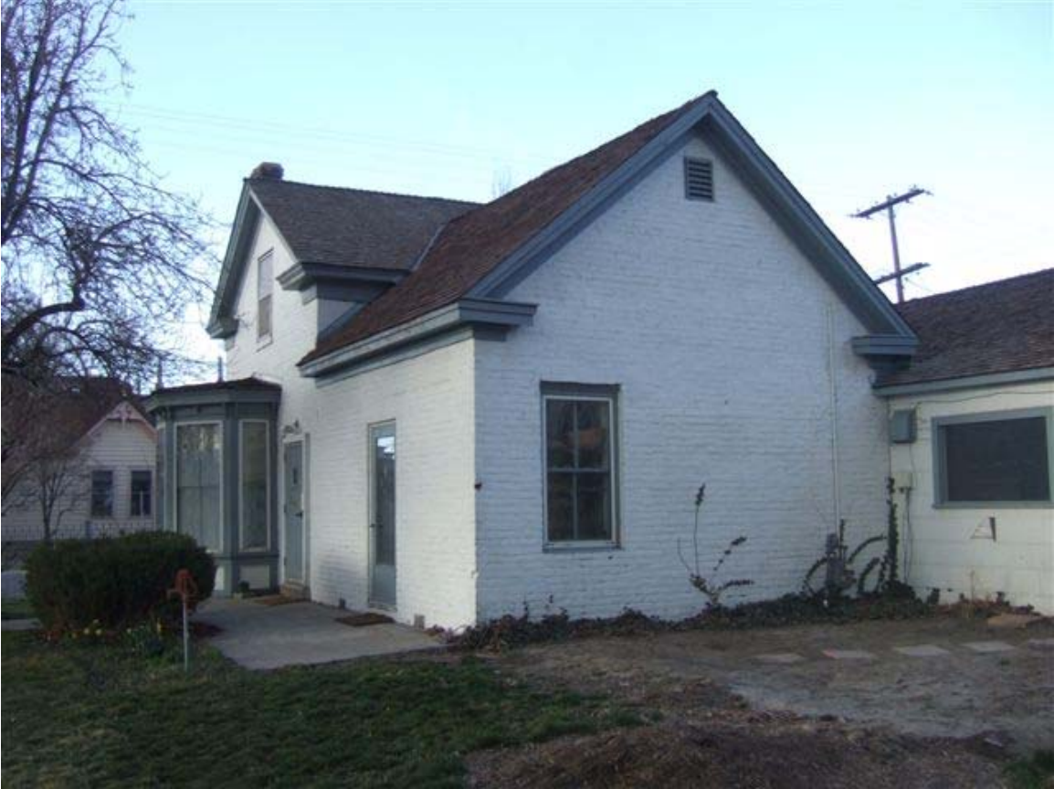
2. East (front) and north elevations of the Rectory.
