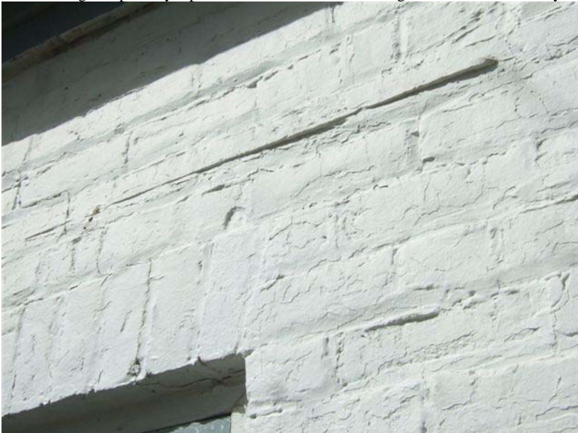
5. Rectory brickwork and front porch evidence (nailers).
